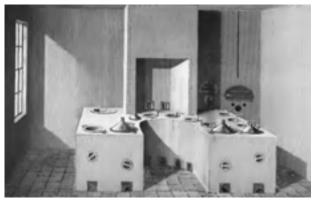
Fig 2. Perspective view of a kitchen fire-place in the house of Baron Lerchenfeld in Munich designed by Count Rumford, ca. 1870
