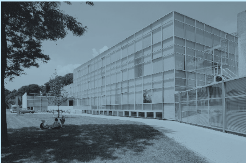
The Rietveld building by architect Gerrit Rietveld houses the Academy of Art & Design and the Academy of Architecture.
